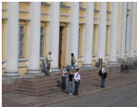
The steps of knowledge. Since 1845 generations of researchers and students have used the collections and research facilities of the university library designed by C. L. Engel. An increasingly larger share of the National Library of Finland's services is being provided through its online services.
